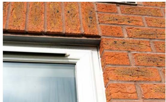
Failed silicon sealant identified and recorded on survey
