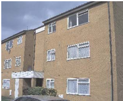
Block of Flats requiring window replacements
