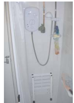
Shower Installation for Disabled Resident
