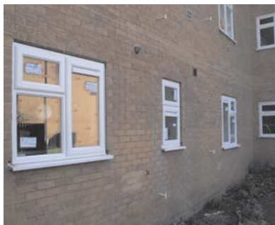
PVC-u replacements in progress
