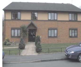
Property on Cyclical Painting and Repairs Programme
