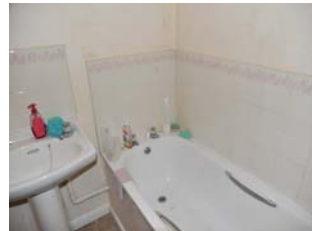
Bathroom (20 years) recorded at Survey
